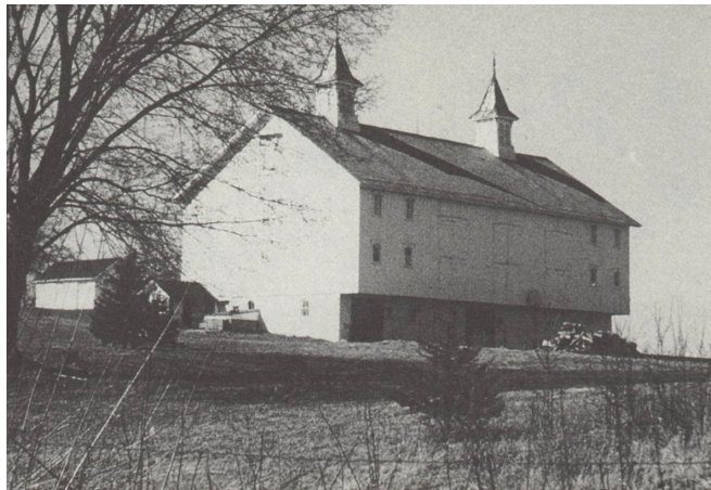
Open forebay Pennsylvania-style barn located in Ohio (photo from Noble and Cleek, The Old Barn Book )
