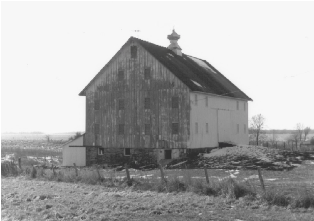
Multi-level gable roof barn (also a bank barn), Midway Stock Farm, Van Buren County, Iowa (National Register photo)
